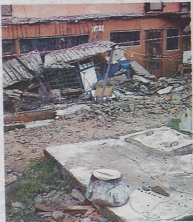
• Collapsed balcony in one of the buildings at FESTAC Extension, Lagos.
