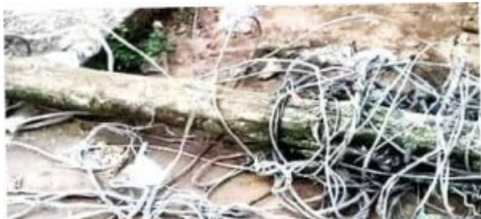
Fallen electric poles and cables
