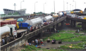
Lagos bridges under threat of collapse from parked trucks
