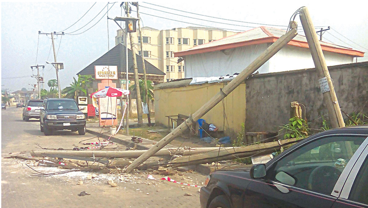
The scene of the fallen electric pole at GRA, Phase 11
