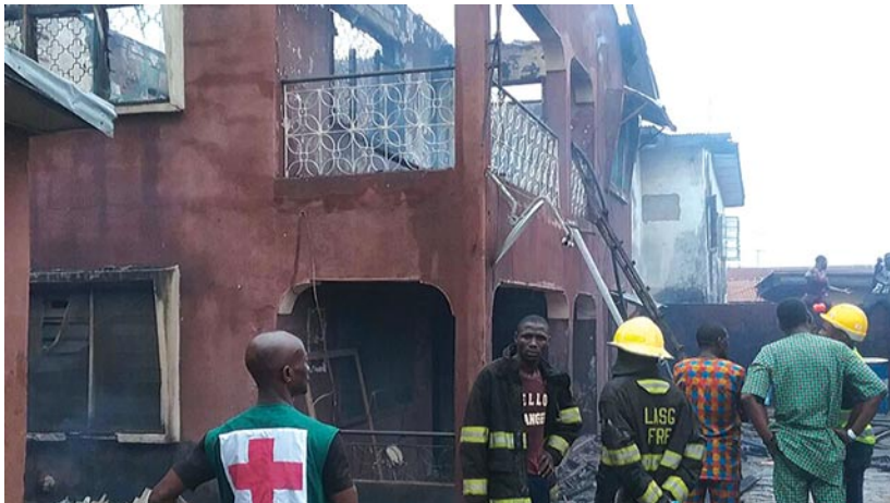
The burnt building
