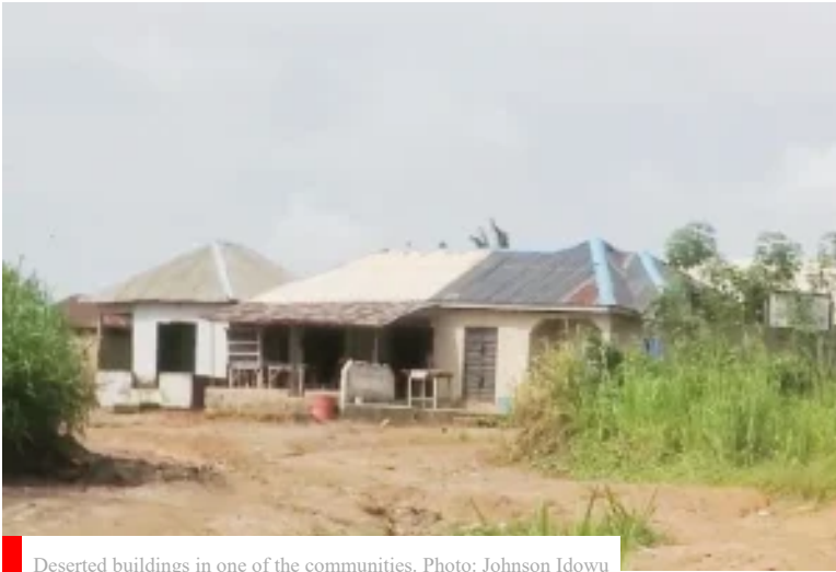
Deserted buildings in one of the communities. Photo: Johnson Idowu
