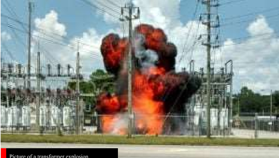
Picture of a transformer explosion
