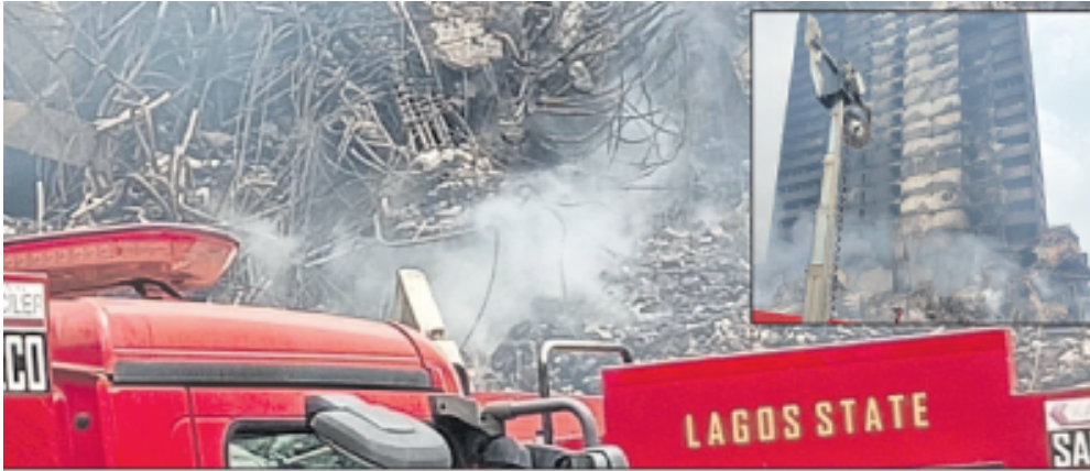
• Fire still burning at GNI Building
